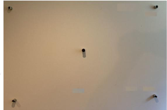
5. Center standoff also takes a flathead set to height so that it is slightly more than height of standoff and spacer. This keeps the board from bowing
