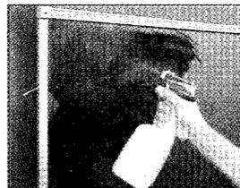
3 Spray a solution of alcohol and water on the surface to lubricate and retard the adhesive.
